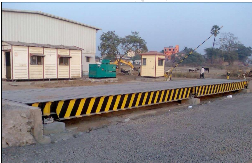
Pit less Weighbridge
